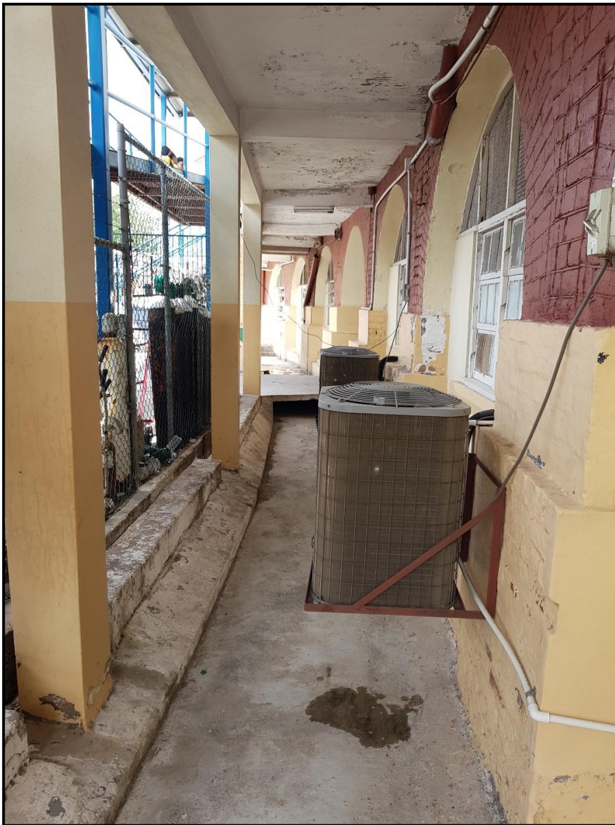
Figure 3. Structural frame of external corridor
